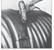
**13** Use a "deep-well socket" and power wrench for rapid assembly. Tap the band during tightening with a rubber mallet to ensure uniform eating of the gasket.
