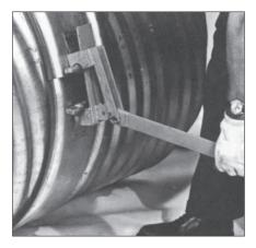
**1** Pull the band into position. For maximum compression of the gasket, the band corrugation must be fully seated into the second corruagtion from each pipe end.
