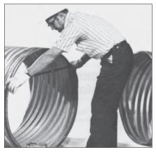
**3** Snap gaskets around and into the first annular corrugation of each pipe end.
