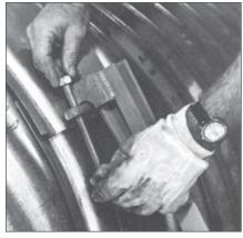
12<sup>Insert bolts</sup> and tighten the band.
