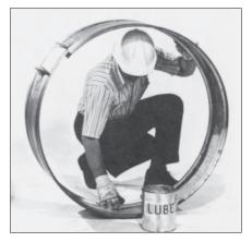
**5** Lubricate the entire inner surface of the band between the corrugations with the same lubricant.
