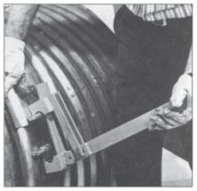
**1 O**<sup>With</sup> the necessary parts lubricated and all foreign matter between the pipe and band removed, use a Felton Puller or long bolt to start the band lap.
