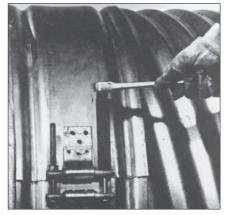
**14** As a guide, torque bolts between 25 to 30 foot-pounds. For maximum compression of the gasket, the band corrugation must be fully seated into the second corrugation from each pipe end. Where specifications restrict infiltration/ exfiltration, a test must be conducted on the assembled joint to confirm proper installation.
