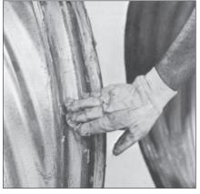
2 Applying additional lubricant to outside pipe ends is not mandatory but is recommended to product optimum results with larger diameters or asphalt-coated pipe in cold weather. Remove any foreign matter that might become lodged between the pipe and the band.
