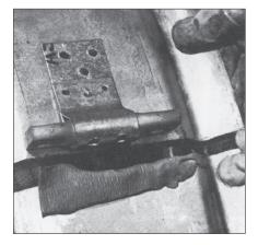
**9** Tuck the mastic over the lip of the band. Note: With double asphalt-coated bands in warm weather (warm enough to cause the asphalt to flow), the mastic may not be necessary. For final determination, use a joint tester to evaluate performance.
